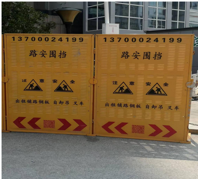
Figure 4. Traditional color steel plate construction enclosure in real-scene use
